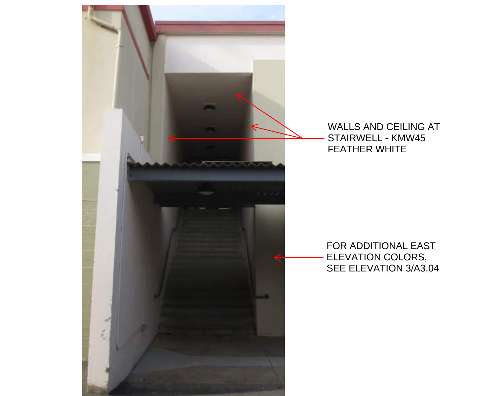
LA BUILDING - EAST STAIRWELLS
