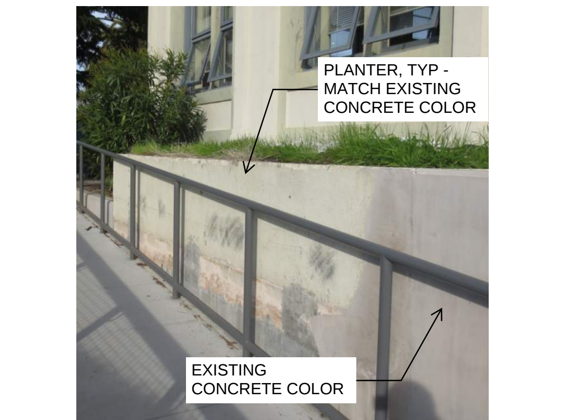
EXISTING CONCRETE COLOR
