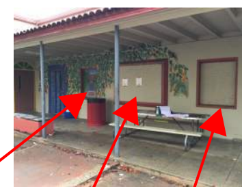
PROVIDE NEW AC PLYWOOD OVER EXISTING OPENINGS - ATTACH TO FRAMES
