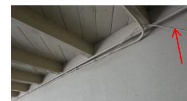
REMOVE COAX CABLING UNDER COVERED WALKWAY. PATCH PENETRATIONS AT WALLS
