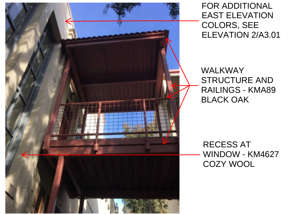
AD BUILDING - EAST WINDOW RECESS AND WALKWAY
