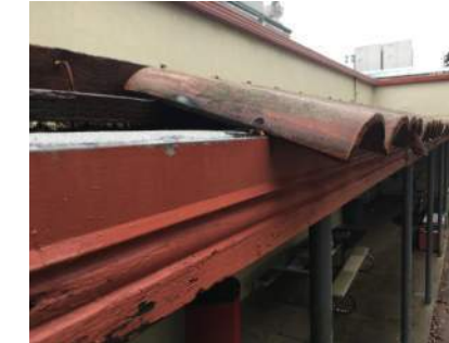
REMOVE SPANISH TILE FROM WALKWAY ALONG TWO SIDES OF BUILDING, REPAIR FASCIA & GUTTER. SEE DETAIL 20/A8.2
