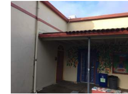
REMOVE SPANISH TILE FROM WALKWAY ALONG TWO SIDES OF BUILDING, REPAIR FASCIA & GUTTER. SEE DETAIL 20/A8.2
