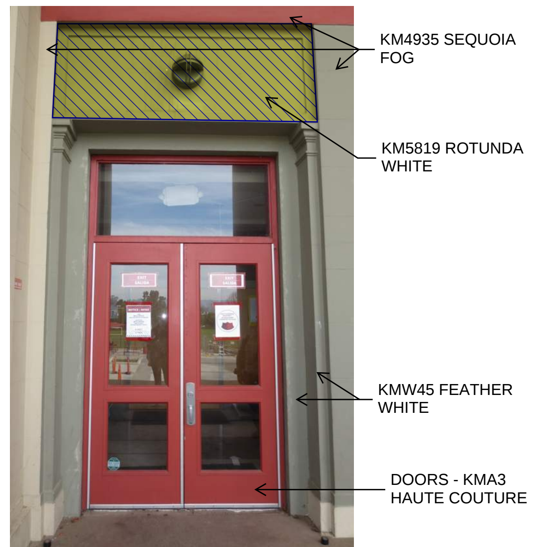
AD BUILDING MAIN ENTRY - FRONT DOORS
